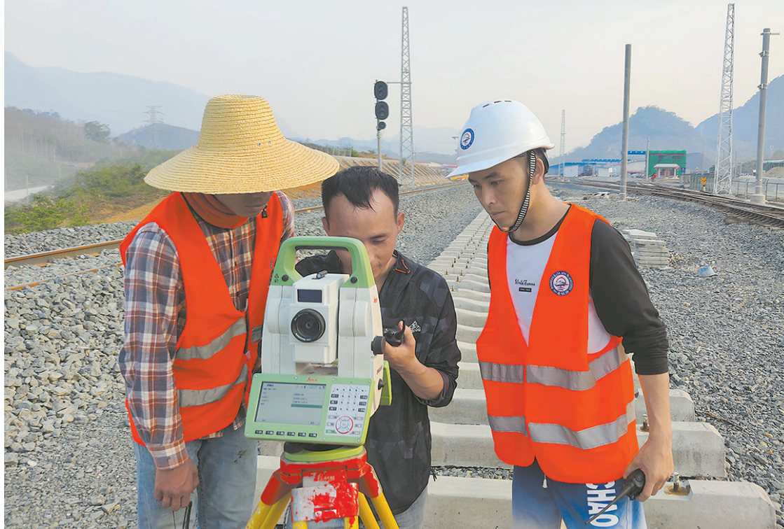
Students learn engineering survey technology at the Luang Prabang railway station on Laos' Mowan section of the China-Laos Railway. — All photos by Ti Gong
